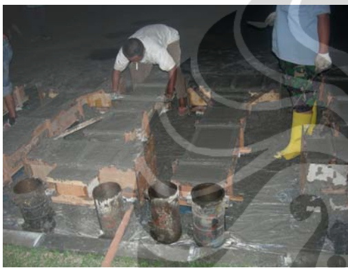
Gambar L49. Finishing
