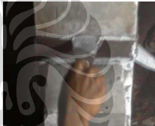
Gambar L101. Pasang Epoxy Pelat
