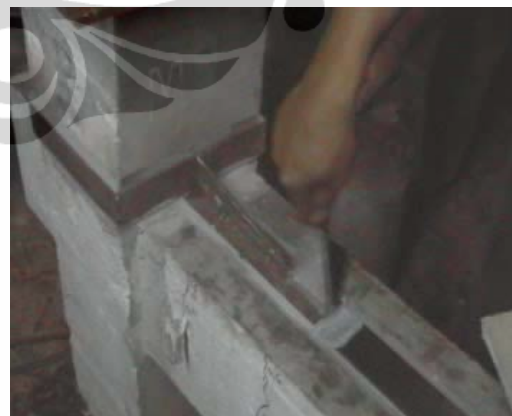
Gambar L103. Pasang Epoxy Pelat
