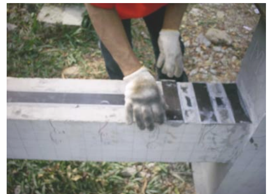
Gambar L97. Pasang CFRP
