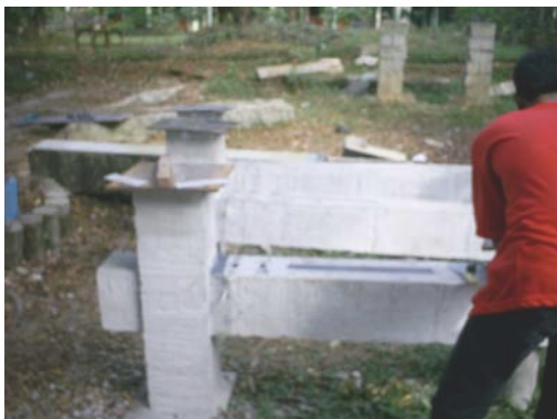
Gambar L96. Pasang CFRP
