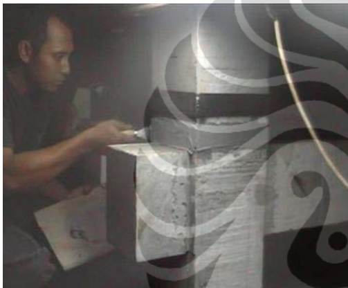
Gambar L100. Pasang Epoxy Pelat
