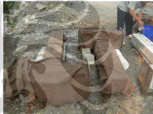
Gambar L55. Proses Curing
