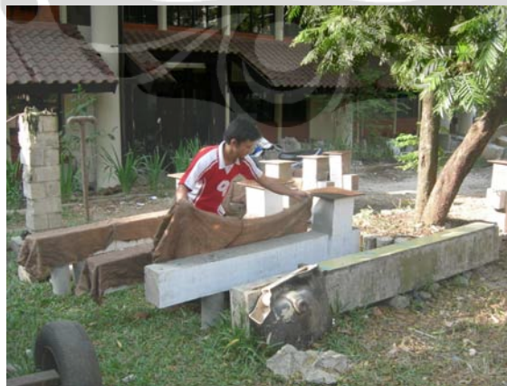
Gambar L56. Proses Curing
