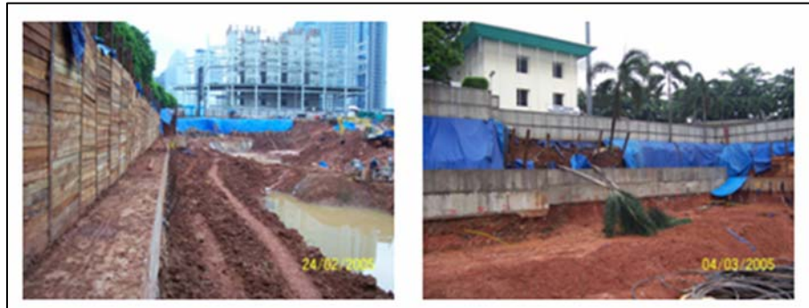
Gambar 5.2 Slope Protection Keliling Galian Pondasi Raft Data Base Kontraktor
