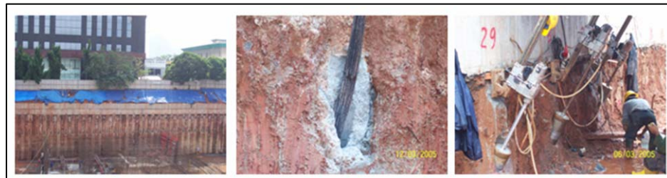
Gambar 5.3 Ground Anchor bersudut 60^\circ (Data Base Kontraktor)
