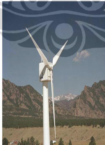
Gambar 2.5 Turbin Angin Sumbu Horizontal
