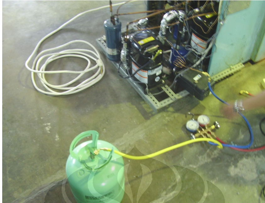
Gambar 3.15 Proses charging R22
