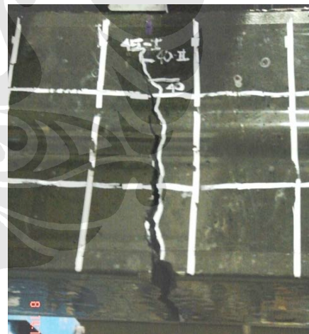
Gambar 4.29 Failure Penampang Balok
