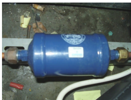
Gambar 3.7 Filter dryer
