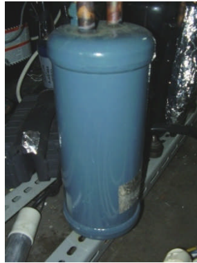
Gambar 3.9 Oil separator
